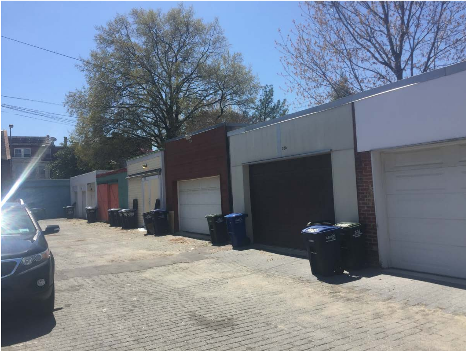
REAR ALLEY LOOKING SOUTH
