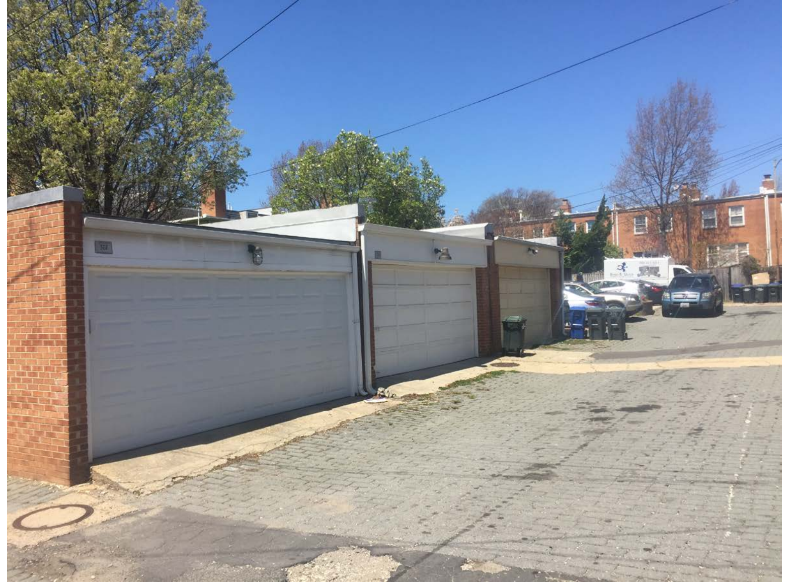
ALLEY, LOOKING NORTH
